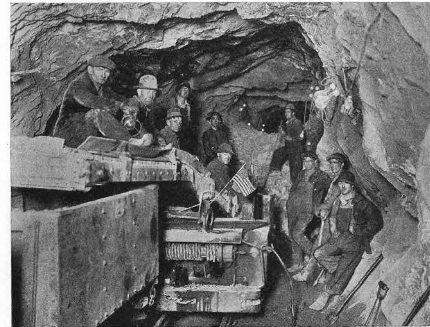
"Mucking Out" the Last Shot in Pioneer Tunnel on May 1, 1928
